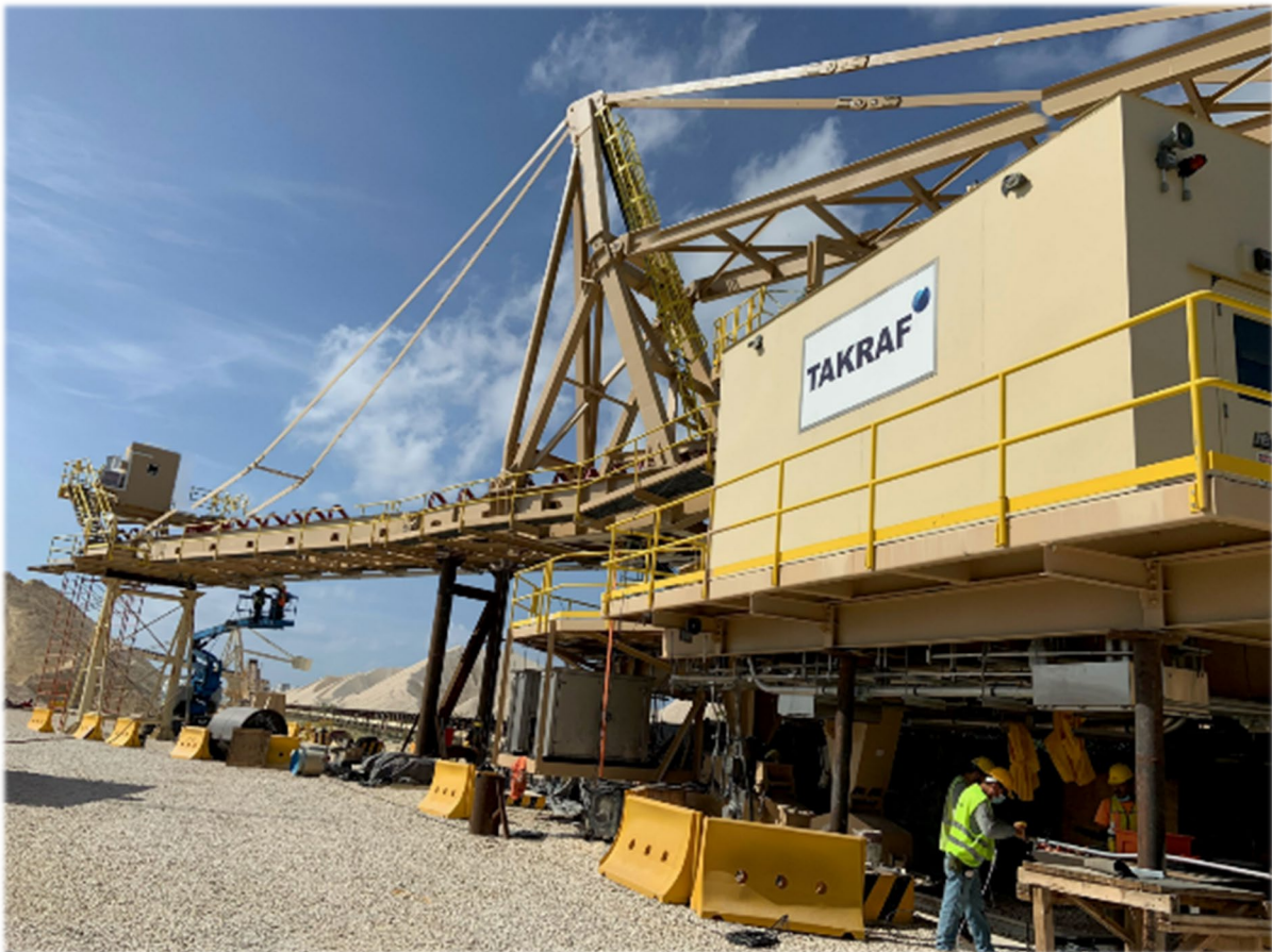
Pic 1: Site erection of the 6,000 t/h TAKRAF stacker in Mexico.
